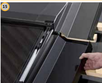
Mount lateral side gutters
