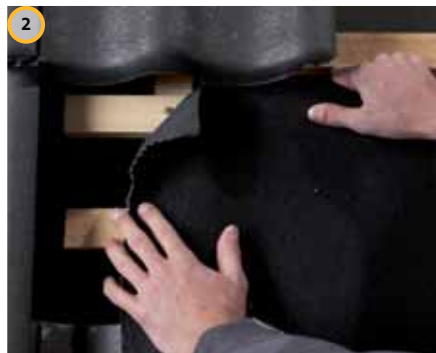
2 Install additional roof laths and mount waterproof skirt
