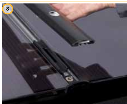
8 Put down laminates and install clamp profiles
