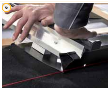
5 Snap rotation anchors into side member and mark fixation point
