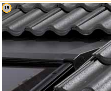
Push the side gutters into the holes of the clamp profiles
