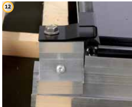
Install protection seal Snap positioning elements LATERAL into the side member profile
