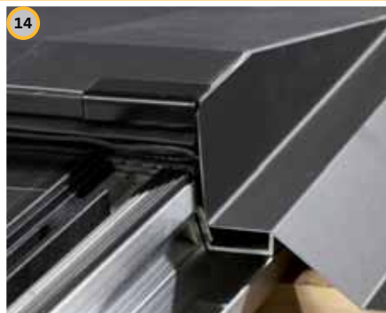
Mount adapters for the upper flashing LEFT and RIGHT
